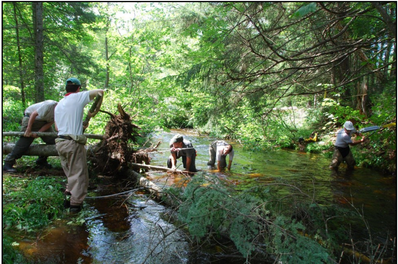
Vermont Fish and Wildlife Department and Trout Unlimited staff constructing a strategic wood addition structure on the East Branch Nulhegan River in northeastern Vermont. Photo Credit: Joe Norton, Trout Unlimited
