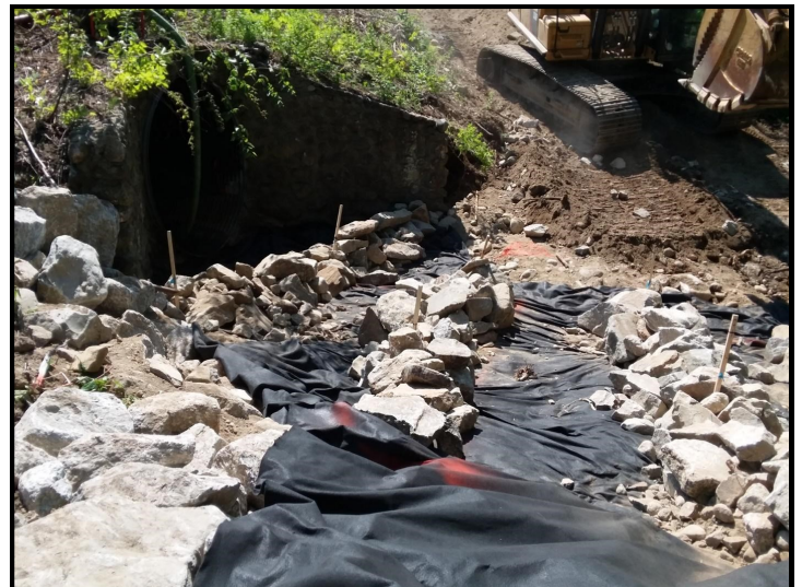
(Top) Placement of fabric and footer rocks at downstream weir. (Bottom) Placement of rubber liner, sand and top band of boulders at downstream weir. The rubber liner was intended to help keep flow on the surface and not go under the band of boulders.
