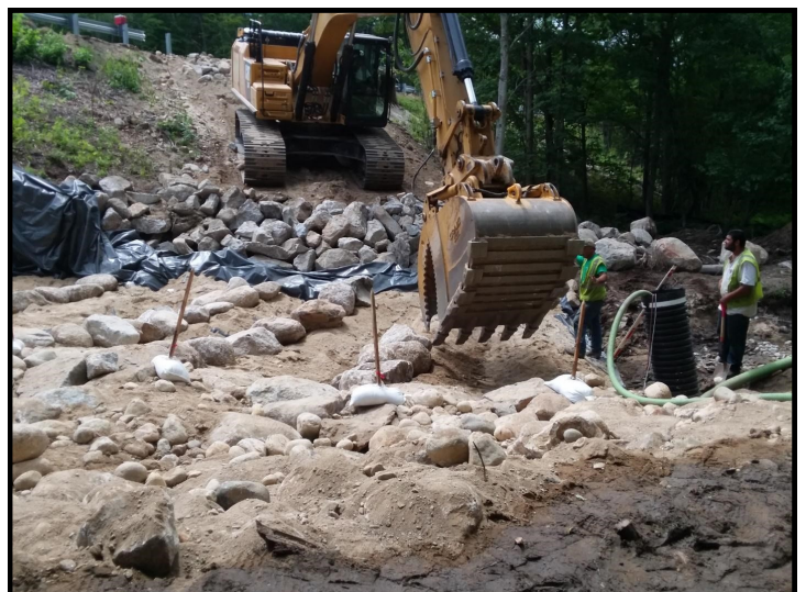
(Top) Placement of fabric and footer rocks at downstream weir. (Bottom) Placement of rubber liner, sand and top band of boulders at downstream weir. The rubber liner was intended to help keep flow on the surface and not go under the band of boulders.
