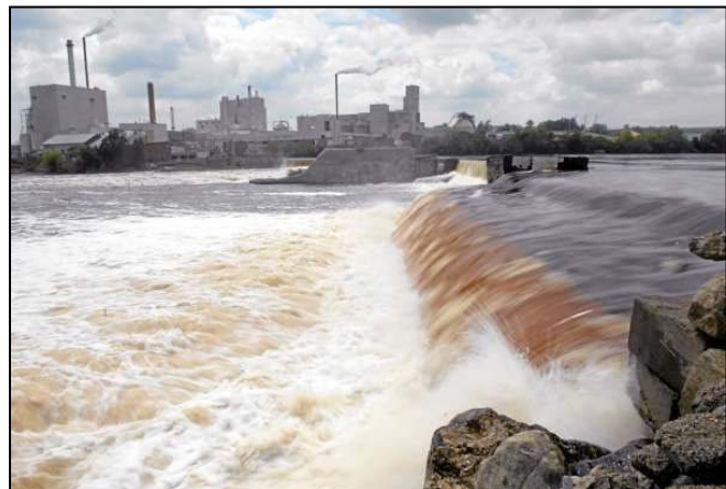
Great Works Dam, viewed from the east side of the Penobscot River
